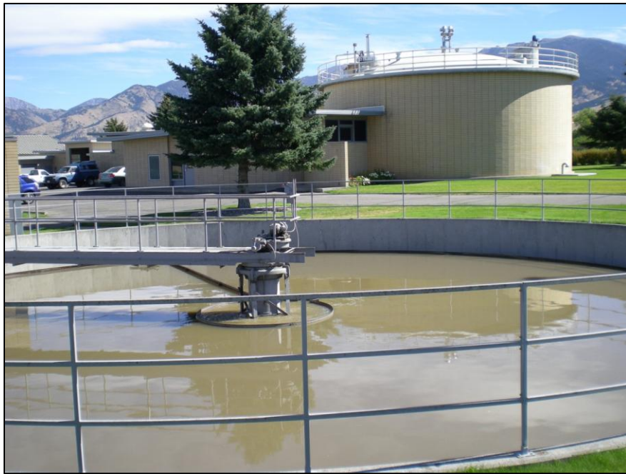
Figure 16. Primary Clarifier Tank at the Bozeman Wastewater Treatment Plant. Incoming wastewater flow is slowed, allowing heavy solids to settle and lighter solids, oils and grease to float to the surface. Scum is scraped off the top and sludge is pumped from the bottom. The remaining water is decanted for continued treatment. (Photo courtesy of Tom Adams)
