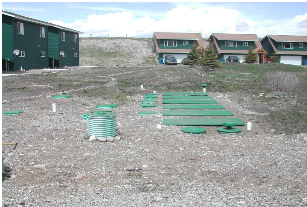
Figure 23. AdvanTex® Level-2 Nitrogen-Reducing Treatment System Installed as Public System. One of seven public sewage systems using recirculating trickling filters. The system is approved for up to 5,100 gallons per day.
