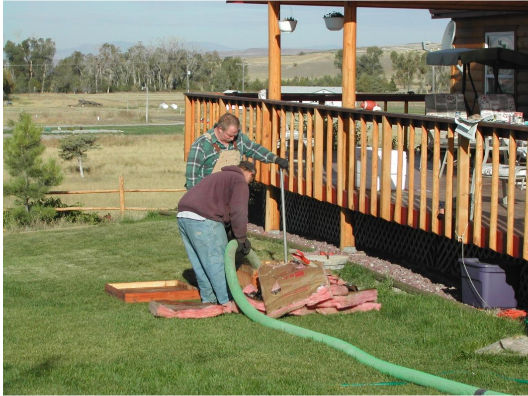
Figure 25. Photograph of a Septic Tank being Pumped. When a septic tank is pumped all of the contents are removed. The combined mixture is called septage, and it includes settled solids (sludge), fats, oils, grease and other floating solids (scum), partially treated wastewater (black water), and any other non-biodegradable trash that has entered the tank (photo courtesy of Alan English).
