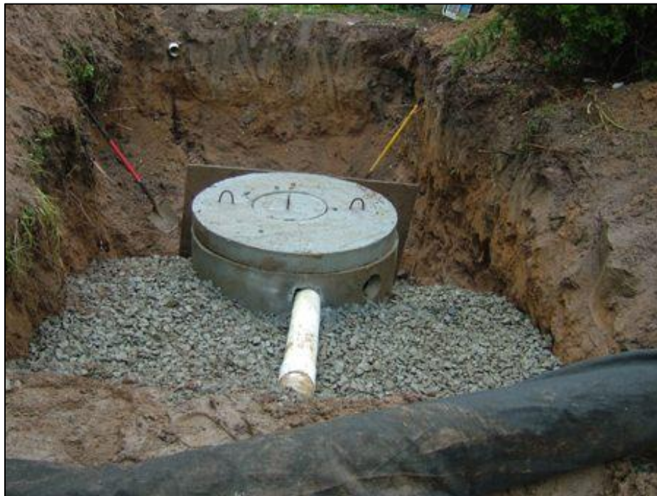
Figure 6. Photograph Showing Installation of a Seepage Pit. The top concrete ring of a seepage pit structure is shown during installation. In this case coarse rock is being backfilled around the outside of the seepage rings. The pipe in lower center is the discharge line from the septic tank.
