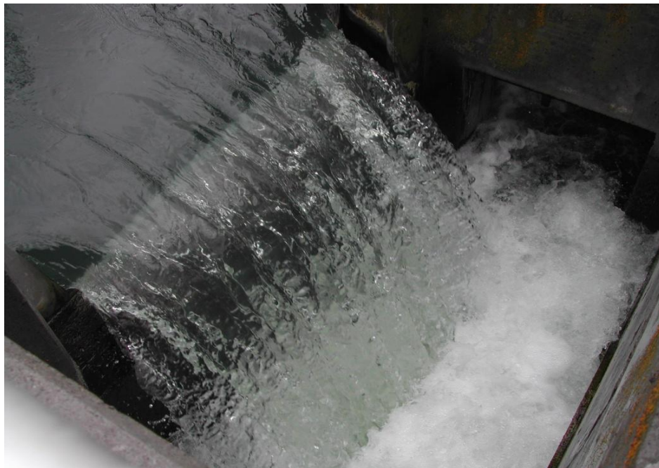
Figure 20. Photograph of Final Treated Effluent Leaving the City of Bozeman Plant. Treated wastewater is disinfected prior to discharge to the East Gallatin River. The structure in the photograph is about 4-feet across, and the discharge is about 5.5 million gpd. Photo by GLWQD
