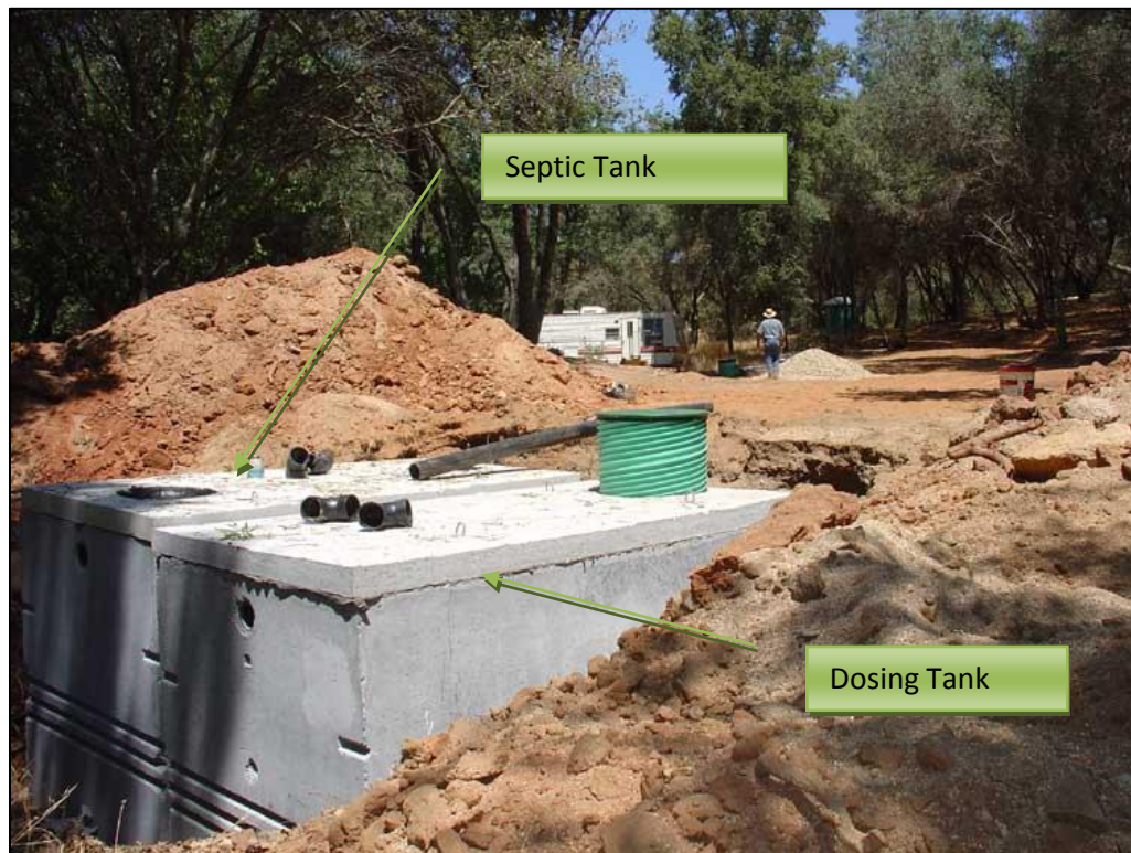
Figure 8. Photograph Showing Installation of a Septic Tank and Dosing Tank. A timer or float controlled pump in the dosing tank periodically pumps effluent to the drainfield under pressure, resulting in even distribution and improved wastewater treatment in the drainfield area.
