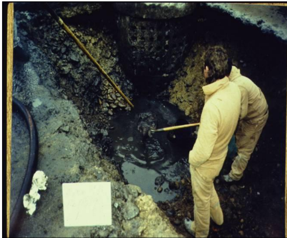
Figure 4. Photograph of a motor vehicle waste disposal well being excavated. Over 100 of these disposal wells were located in Missoula, and closed by EPA. Many of them required extensive remediation. In this photo soils around the dry well (top-center) are heavily contaminated with motor oil and solvents. Photograph courtesy of the Missoula Valley Water Quality District.
