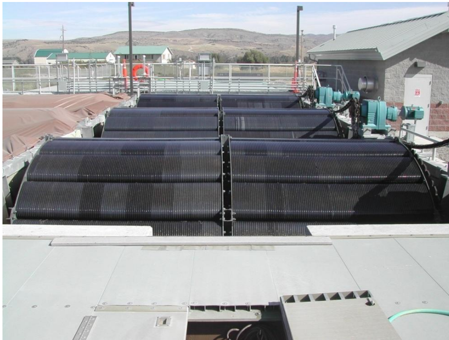
Figure 17. Biowheels at the New Manhattan Wastewater Treatment Plant. The biowheels provide a substrate for bacteria and protozoa that treat the wastewater to colonize on. The biowheels slowly rotate in the wastewater providing contact with the bacteria and protozoa, and aeration of the wastewater.
