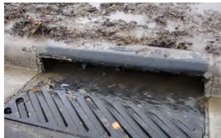
Sediment and other contaminants enter a storm drain during a rain event.
