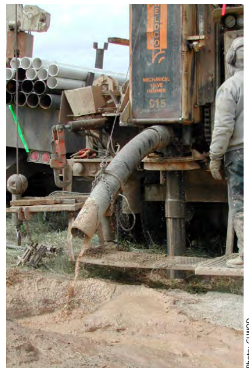
Drilling a domestic well.
