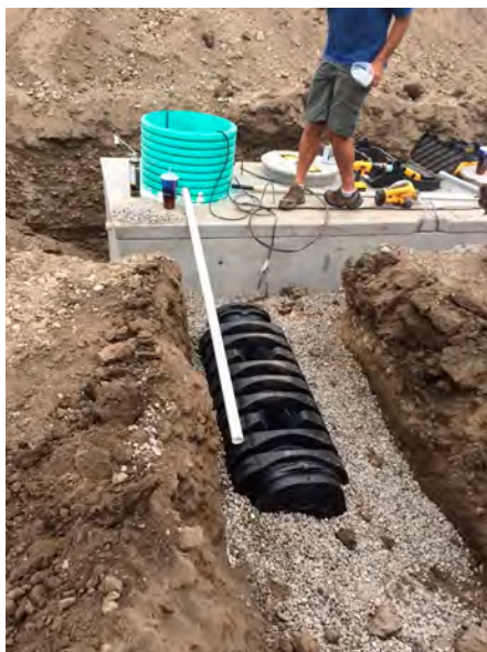
Installation of a septic system.
